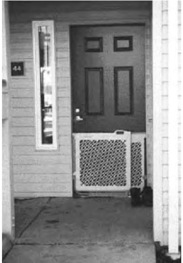
Fig. 1. The child's safety gate illustrates the need for further development of the lever door handle to be fully universal in a family housing setting.
