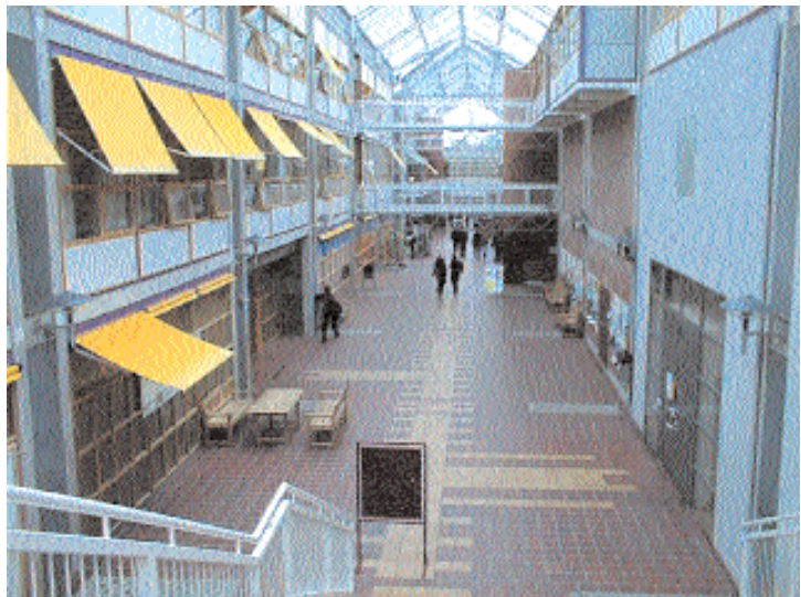
Fig 1. Glazed "street" at Dragvoll University Centre.
